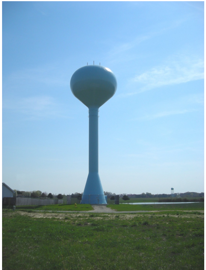
Worton Butlertown, 250k Gallon EST, Kent County, MD.
